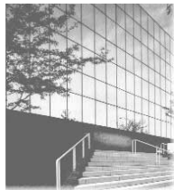
ALL THAT GLITTERS is gold. 22,000 square feet of gold-toned glass helps reduce heating and cooling costs, saves fuel, and makes optimum use of daylight illumination.
